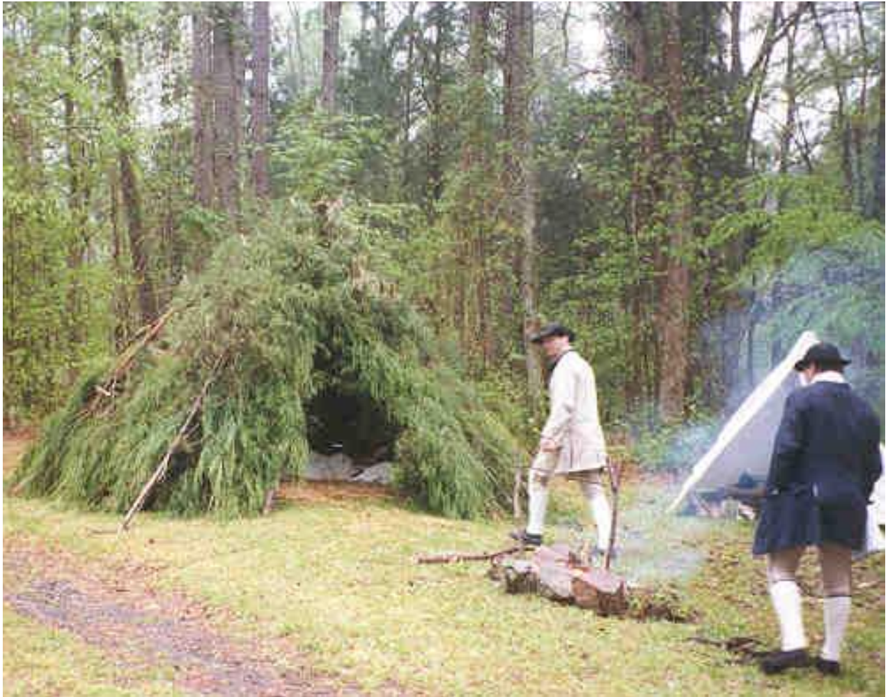
One form of brush hut (wigwam) likely constructed by British and Continental soldiers. After erecting a tripod of long poles (tied together at the top), additional poles are added to fill in the structure, and leaf-covered branches or pine boughs placed over them as a covering. (Photograph by John Rees, North Carolina Volunteers, Historic Stagville, April 1997.)
