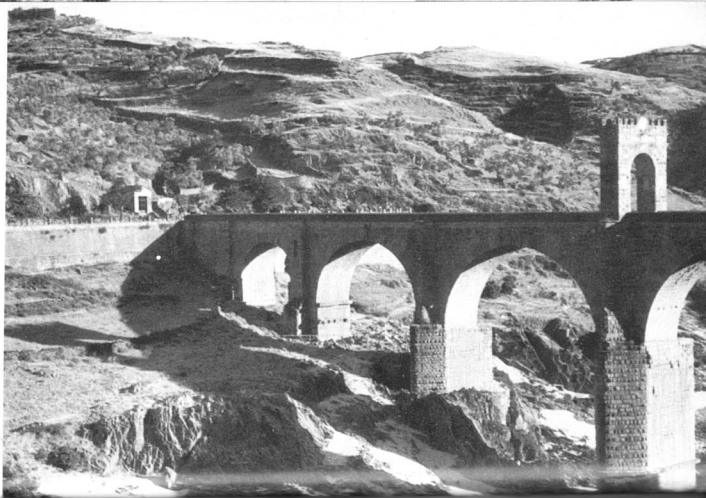
10. The Roman bridge across the Tagus at Alcantara. After being blown up early in the war, it was kept in operation by a simple form of suspension-bridge.
